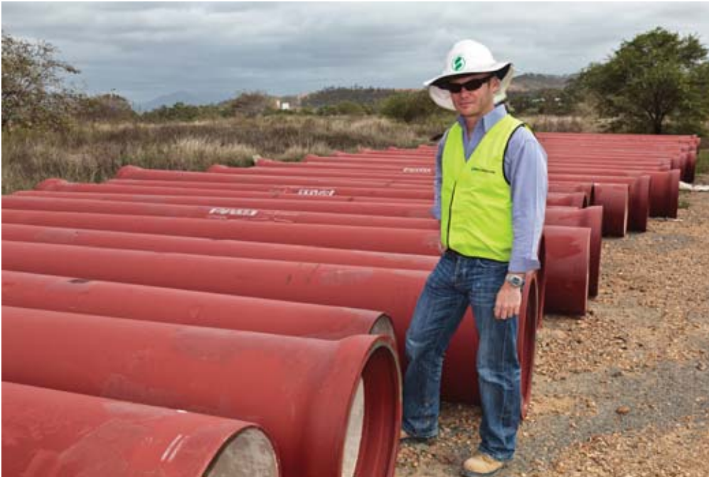
Main: Baulderstone's with 600DN Sewer Ductile Iron Pipe. Top: Vinidex & Baulderstone staff with PE pipe and Vinidex Supermain® PVC-O. Top: 2nd Construction of pipe system. Bottom: Vinidex polyethylene pipe.
