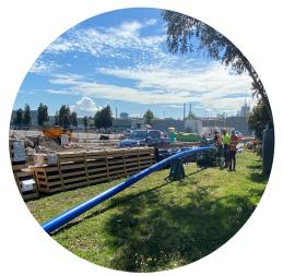
Installation of 400m of DN180 Protecta-Line<sup>®</sup> pipe was completed in November 2020. "Installation was like regular PE pipe, it was easy to use and easily adaptable where existing services or obstructions can affect the proposed alignment." - Winslow Group. It was also ideal for sleeved applications. The only extra attention required was the wrapping of joints and slightly more care required during handling and installation.
