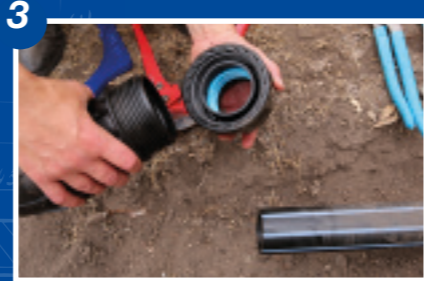
3 Take the fitting apart, remove the nut.
