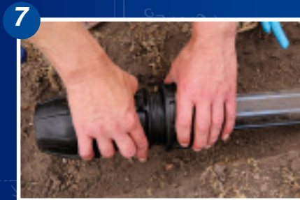
7 Tighten the nut by hand.
