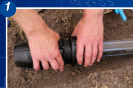
1 Use the multi-grips to loosen the nut then continue to loosen by hand and slide the body off the pipe.
