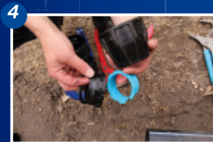
4 Remove the split ring and collet, ensuring you keep them together. Remove the O-ring.
