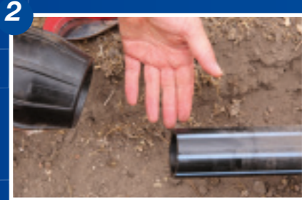
2 Cut the pipe square. There is no need to chamfer or lubricate the pipe.
