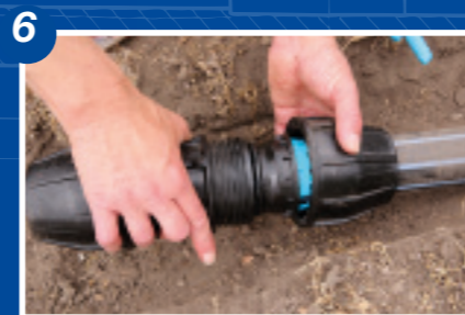
6 Insert the pipe into the fitting body ensuring pipe butts against tapered wedges in body of fitting. Bring the components up to the fitting body.
