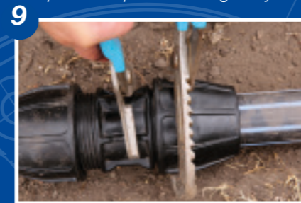
9 The fitting is now fully installed
