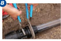
While holding the body tighten the nut all the way to the flange using multi-grips
