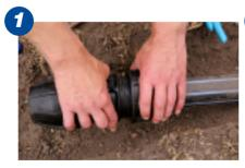
Use the multi-grips to loosen the nut then continue to loosen by hand and slide the body off the pipe.
