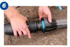
Insert the pipe into the fitting body ensuring pipe butts against tapered wedges in body of fitting. Bring the components up to the fitting body.
