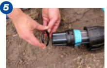
Slide the components onto the pipe, first the nut, then the split ring and collet followed by the O-ring.
