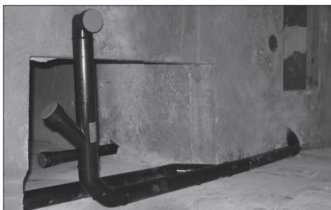
Illustration 9.2 Prefabricated pipe sections installed on site
