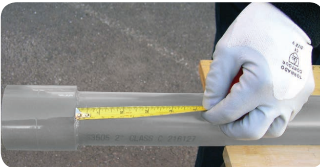
8. Using the mark previously made, check that the pipe has been fully inserted.
