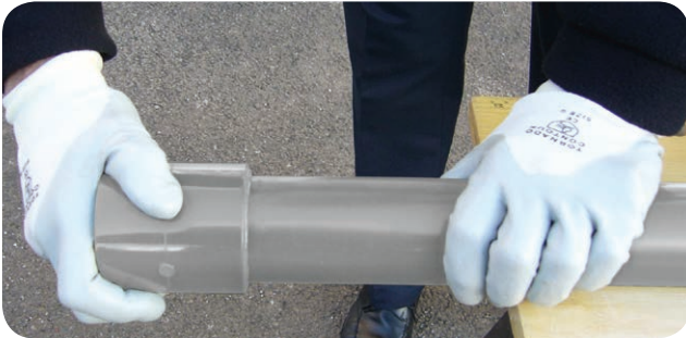
7. Wipe off excess cement from the outside of the joint.
