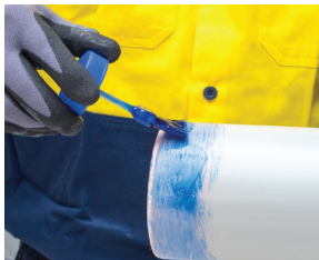
Pressure applications using Vinidex Type PSolvent Cement.
