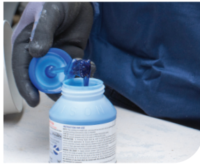
For larger pipe diameters a larger brush should be used.
