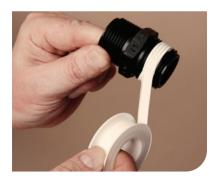
1. Apply PTFE tape or approved sealant to the male thread the blue handled ball valve is to be screwed in too. Sufficient tape needs to be applied to ensure a watertight seal
