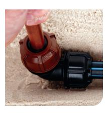
4. Insert the copper pipe and push into the rubber seal up to the mark indicator
