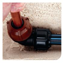
5. Tighten the nut by hand and finish using a wrench. Remember to check that the nut is tight against the body flange.
