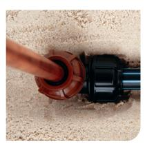
6. Remember to replace the stainless steel grip ring if re-using the copper connection.
