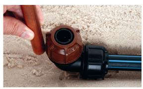
3. Cut copper pipe square. The fittings is pre-assembled and ready to use. Mark the depth of copper insertaion using 'pipe stop' marking or body flange as visual indicator. Remove any scale or burrs from the copper pipe.
