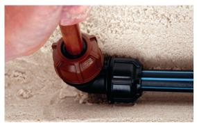
5. Tighten the nut by hand and finish using a wrench. Remember to check that the nut is tight against the body flange.
