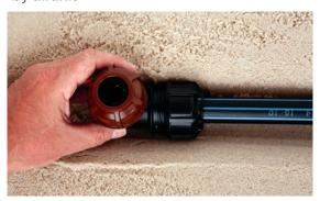
Cut PE or poly pipe square and insert until pipe stop is felt.
