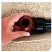
2. Tighten the nut by hand ensuring the nut flange is touching the fitting body, use a wrench if neccessary.
