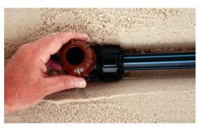
2. Tighten the nut by hand ensuring the nut flange is touching the fitting body, use a wrench if neccessary.
