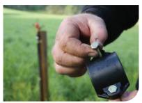
2. Insert the bolts into the saddle bottom and push firmly into the hex recess.
