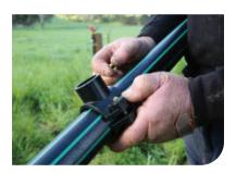
4. Thread each nut onto the bolt until firm and then complete tightening with a spanner.
