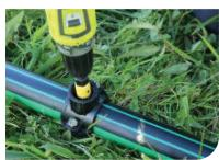
Drill a hole using the correctly sized drill bit taking care not to damage the seal or thread.
