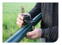
3. Assemble the saddle halves in the desired location on the Rural poly pipe.
