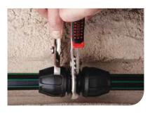
6. After tightening by hand please tighten nut a further 1/4 turn using a wrench.
