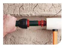
3. Place the insert in the pipe and knock in fully using a blunt object (a soft hammer or piece of timber is ideal) until the pipe end abuts the insert flange.
