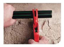
1. Cut the pipe square (preference is with pipe cutters as a hacksaw can leave burrs which require removal).
